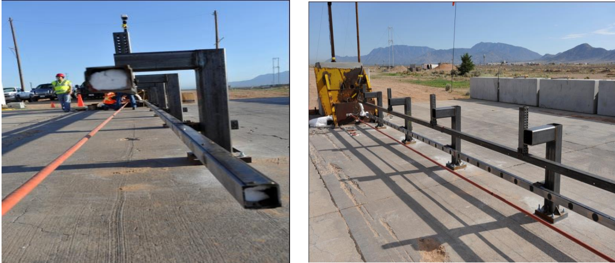
Figure 2. Thermal rails and insulated tow rope in place
